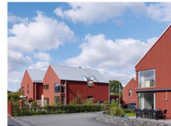
Villor (Sweco Architects)
