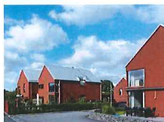
Villor (Sweco Architects)
