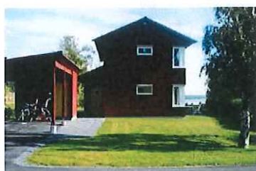
Villor (Sweco Architects)
