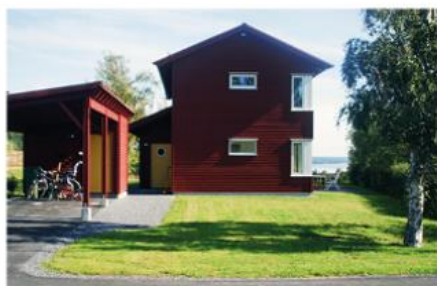
Villor (Sweco Architects)
